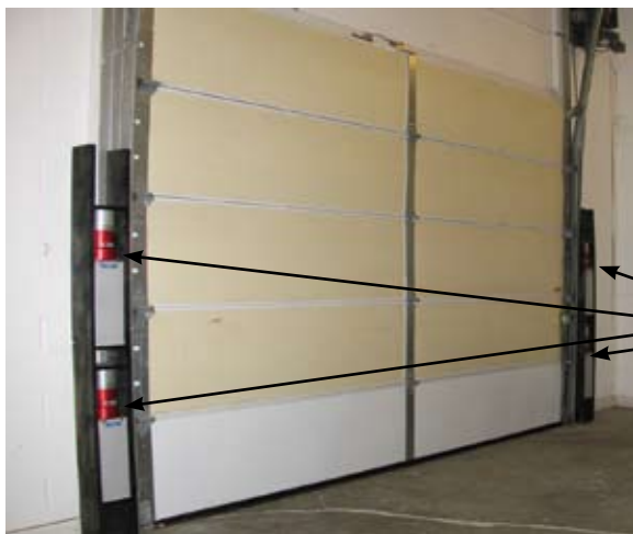
The photo on the left shows four "bars" mounted on a loading dock door.
